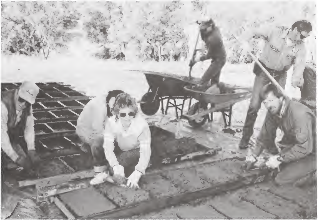
Figure 28. Kentucky Camp workday in 1992 -- Forest employees making adobe blocks. Photo by Jim McDonald.
